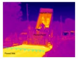
In this thermograph, ten points on the paved mat were selected about 5 feet behind the paver. The difference between the highest temperature (244.6°F) and the lowest temperature (236.6 °F) is only 8°F, which is well within the Georgia state requirement of 20°F. The mat shown was laid by a train that included a remix paver.
